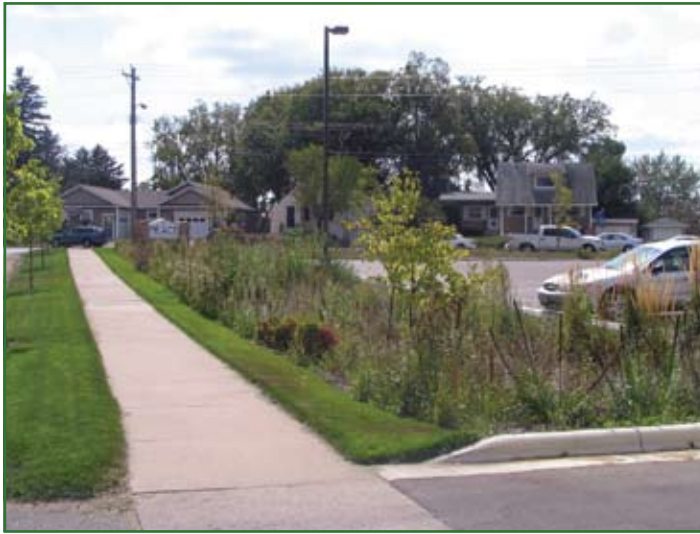
The Peace Church parking lot expansion project included a large-scale “infiltration” raingarden using native plants and grasses to capture storm water runoff.
